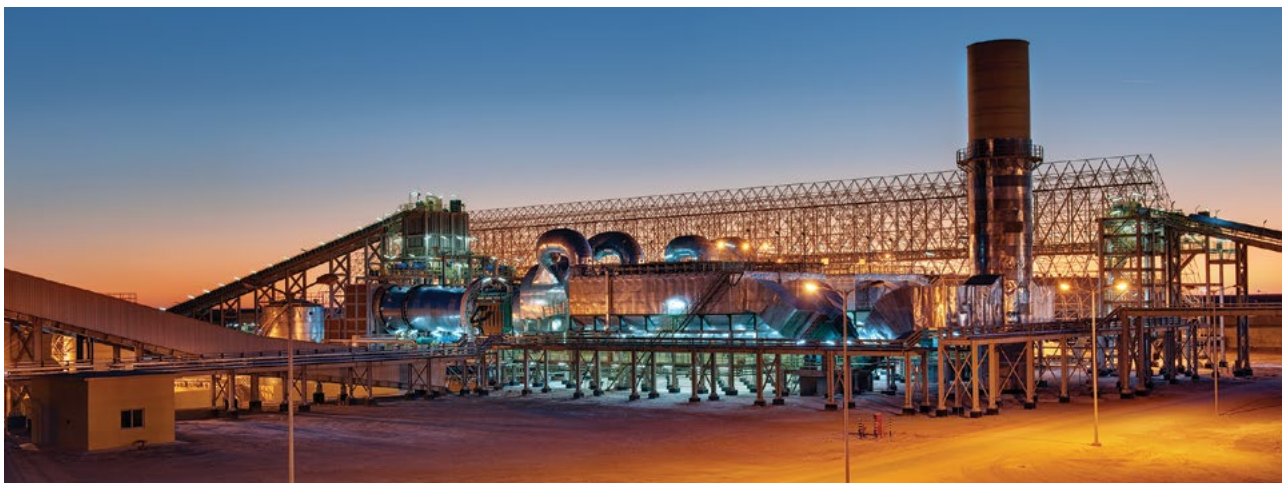
Ma’aden Phosphate Plant - Al Jalameed
